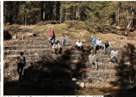
Hidden Creek Restoration completion October 2015.
