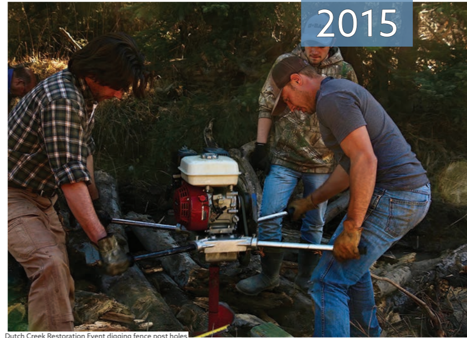
Dutch Creek Restoration Event digging fence post holes
