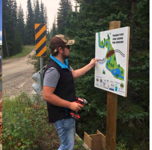
Installing a “Thank you for using the bridge” sign next to Dutch Creek.
