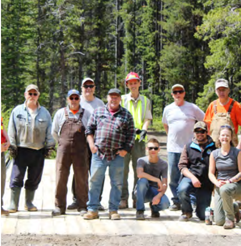
Helping re-deck a bridge over Allison Creek at Ed Gregor Memorial Stewardship Day. Photo Credit: Crowsnest Pass Quad Squad
